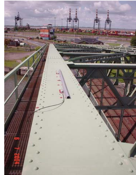
Optical Strand on main bearing on road side
