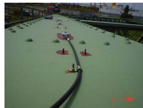
Special welding fixations of the Optical Strand on the beam
