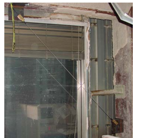
Optical Strand on the underside of the 15 th floor
