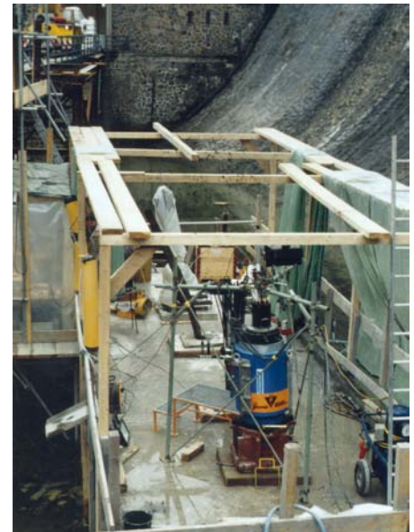
Apparatus equipped with vertical hydraulic jack for tightening tension rods
