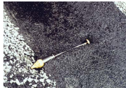
Concrete/asphalt junction of the extensometer
