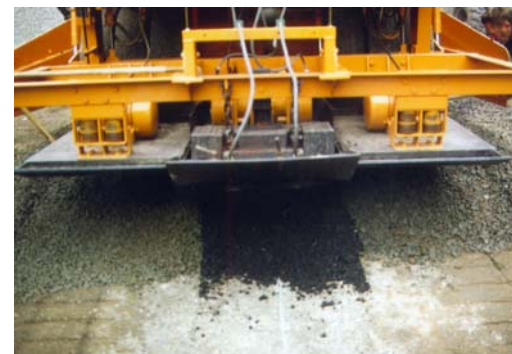
Positioning of an asphalt seal
