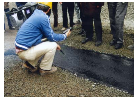
Checking the quality of the asphalt
