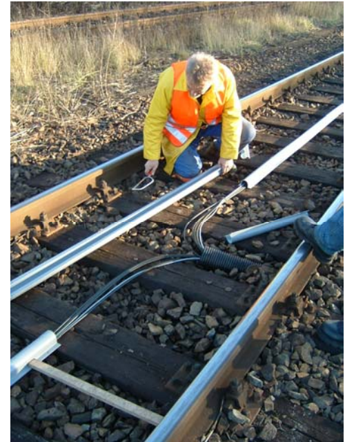
Optical Strands installation on the track
