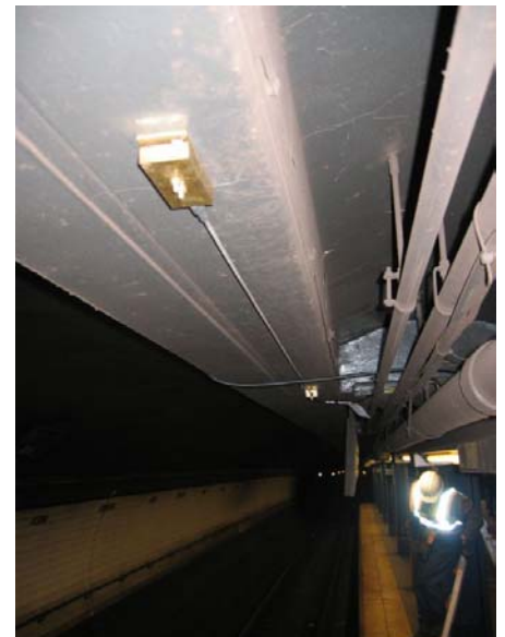
Optical Strand on a beam
