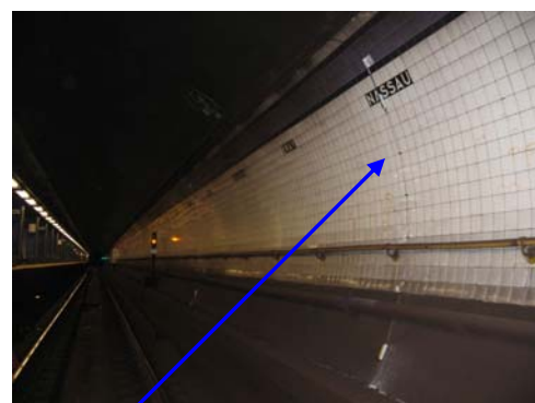
Optical Strand on the tunnel vault
