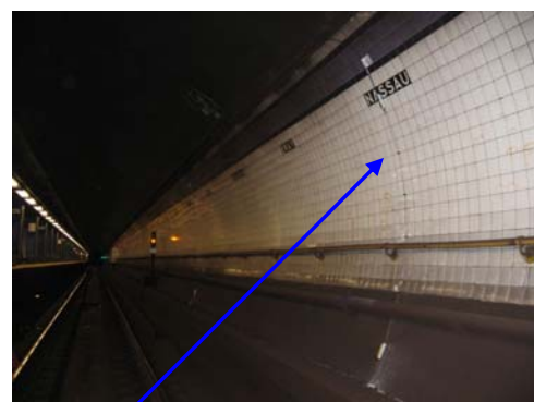
Optical Strand on the tunnel vault
