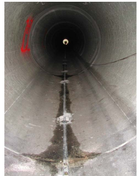
Optical Strand on the pipe
